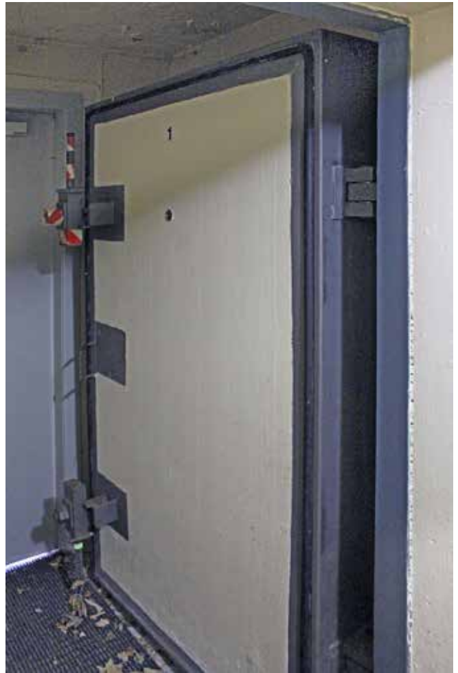
Interior view of reinforced concrete blast door at main entrance
